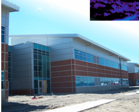
(photo above) Thermographic imaging displays the excellent energy efficiency performance using insulated precast wall panels with edge-to-edge insulation.
