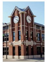
The new Salin Bank building in downtown Fort Wayne, IN needed to reflect its historic surroundings. In order to accomplish this, the architect, MSKTD & Associates, Inc. of Fort Wayne, chose architectural precast concrete. By using architectural precast concrete the architect received the color uniformity and design freedoms desired while using the precast in a structural capacity as well. The Precaster assisted the architect with detailing, color
