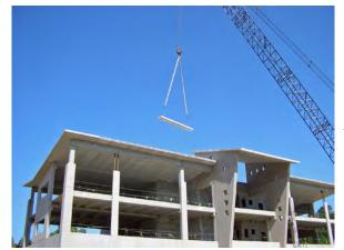
Riverfront Professionals Office Building, located on the Tennessee River in Chattanooga, is a three story, precast structure consisting of Architectural Wall Panels, precast beams, girders and 8" prestressed hollow core panels. The building, constructed by The Strauss Co. is currently in the process to receive certification as a LEED NC Silver facility.
