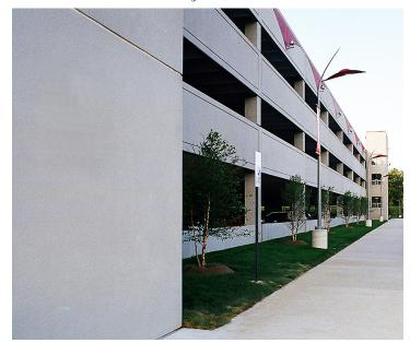
"We selected precast for the Firekeepers Casino Parking Deck because of the tight schedule and winter construction. The ability to erect through the winter months allowed the project to be completed on schedule. Precast also resulted in an initial lower cost."
